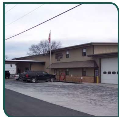
Fairfield Community Fire and EMS Facility, Fairfield Borough
