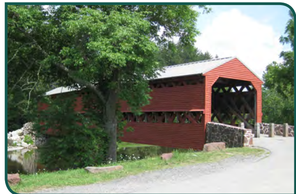
Sach's Covered Bridge, Freedom Township
