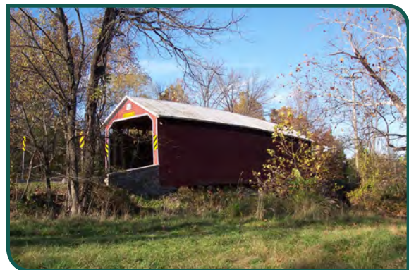
Jack's Mountain Covered Bridge, Jack's Mountain Road, Carroll Valley Borough
