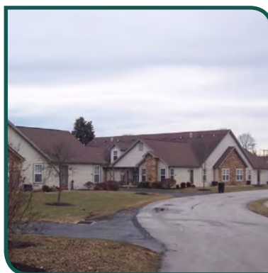
Meadowbrook Commons, Fairfield Borough
