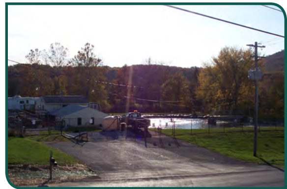
Carroll Valley Sewer Plant, Sanders Road, Carroll Valley Borough
