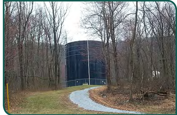
Fairfield Municipal Authority Standpipe, Iron Springs Road, Hamiltonban Township
